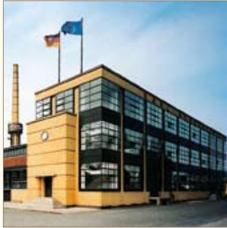
Fagus Factory, constructed by Walter Gropius in 1911
